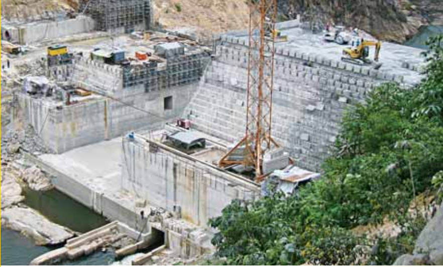
Left – Construction of the US$53 million 19-MW Vaca hydroelectric generating facility on the Macal River in Belize is scheduled for completion at the beginning of 2010. Right – Fortis Generation has a combined generating capacity of 195 MW, 190 MW of which is hydroelectric generation.
