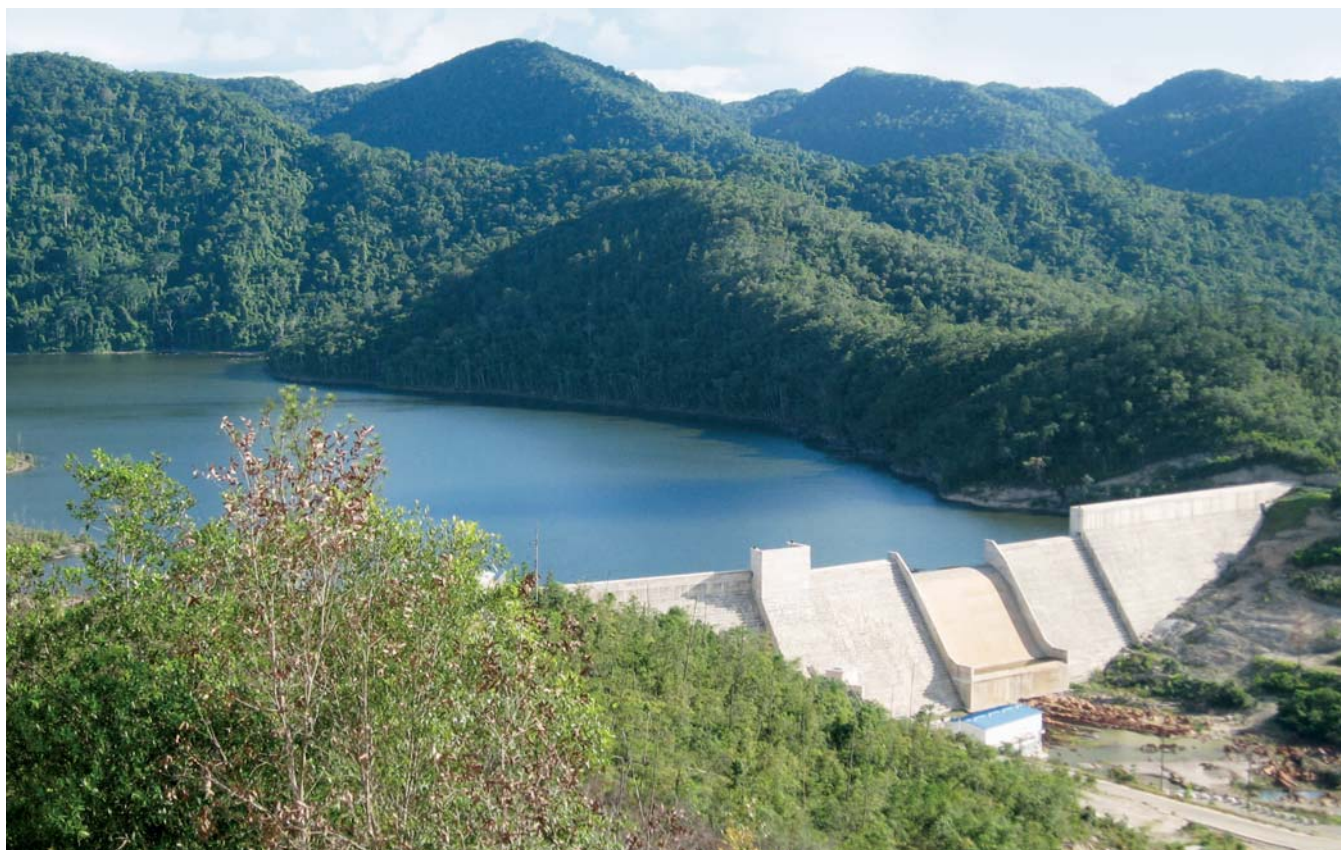
Fortis Generation includes the operations of non-regulated generating assets in Belize, Ontario, central Newfoundland, British Columbia and Upper New York State. The generating capacity of these assets is 195 megawatts ("MW"), 190 MW of which is hydroelectric generation.
