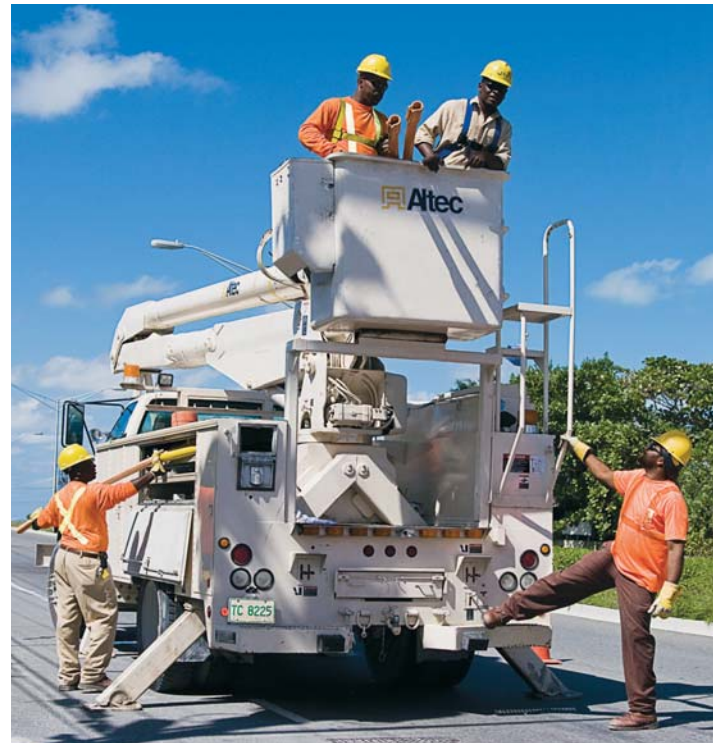
Fortis Turks and Caicos has a combined diesel-fired generating capacity of 48 MW and met a combined peak demand of 28 MW in 2007.
