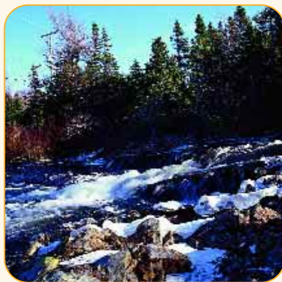
FortisUS Energy operates four hydroelectric generating stations.
